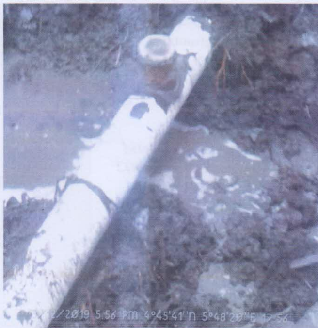
Fig C: Incident facility during repairs
